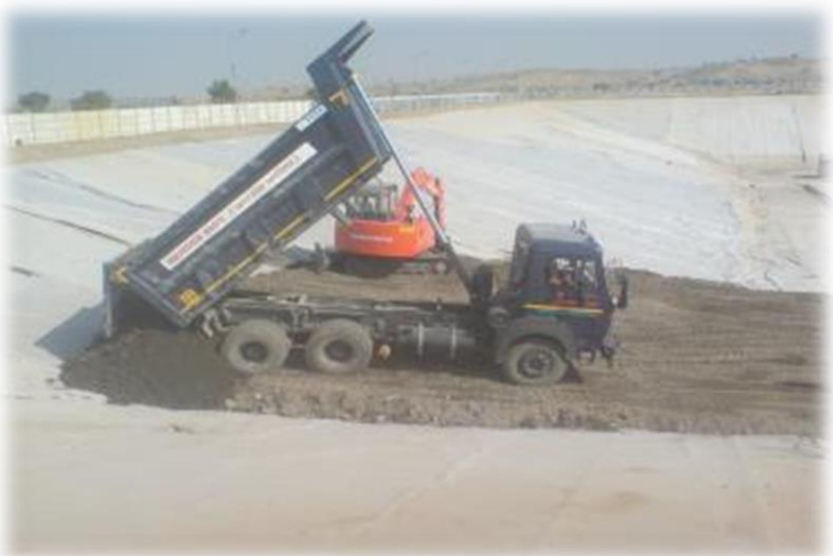
Captive Hazardous waste (double composite liner) landfill
