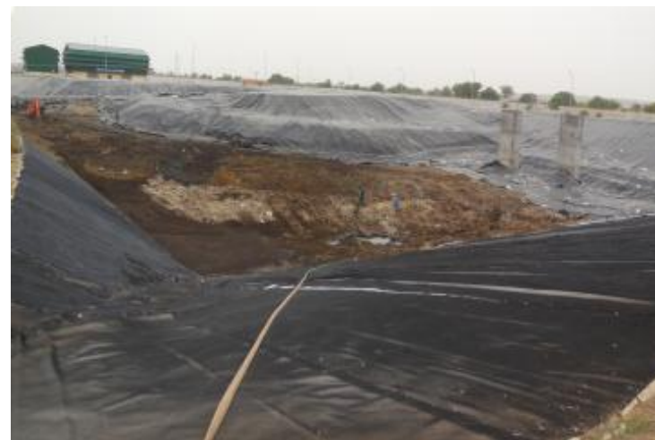
Landfill image taken after capping
